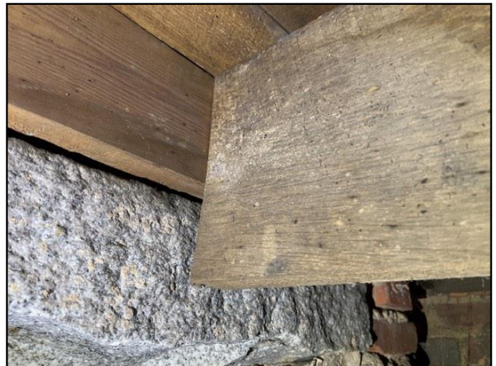
169. Poor end bearing, joist hanger connections
