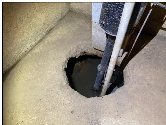
251. Lid missing, rotted or not secure
