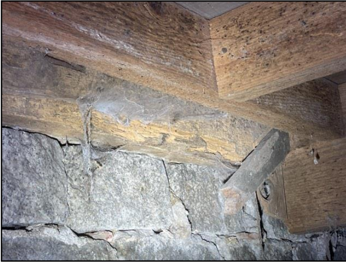
159. Evidence of wood destroying insects.
