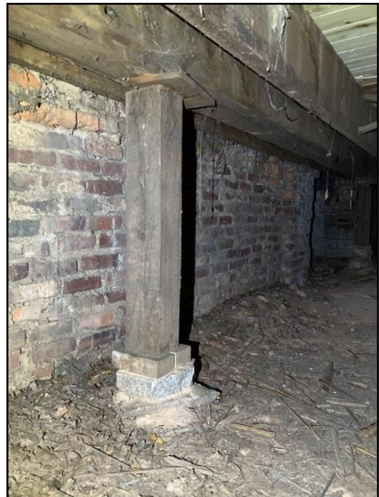
140. Poorly secured footing
