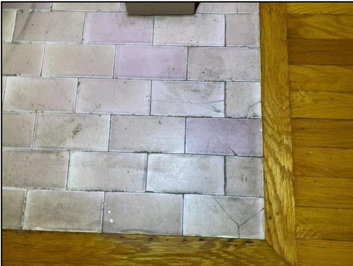
234. Gaps or cracks
