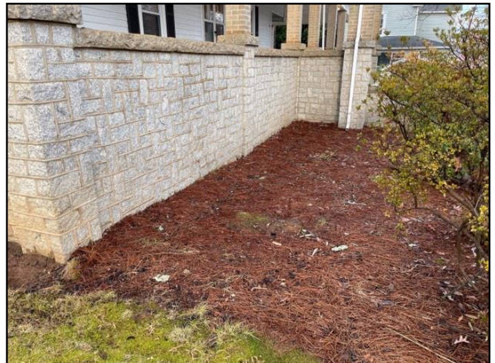
79. Improper slope or drainage
