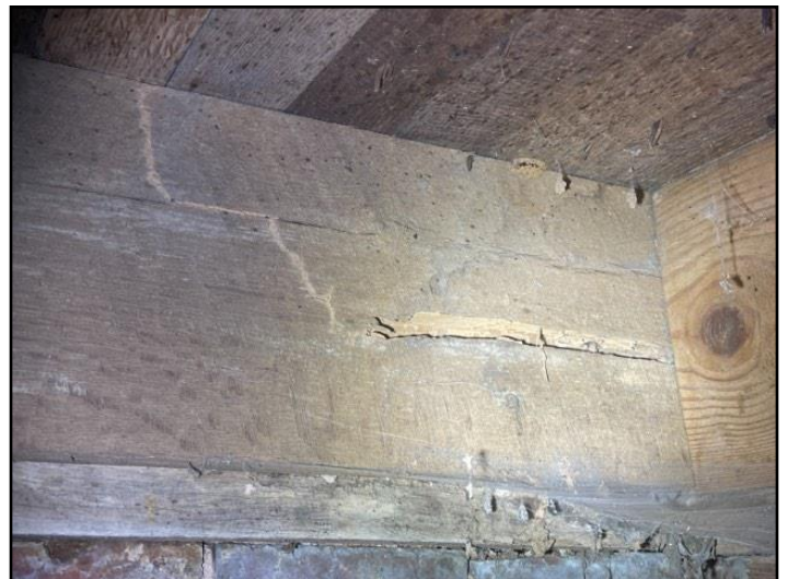
158. Evidence of wood destroying insects.
