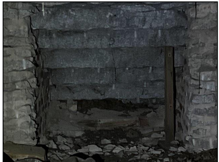
65. Inadequate support for stair - stair...
