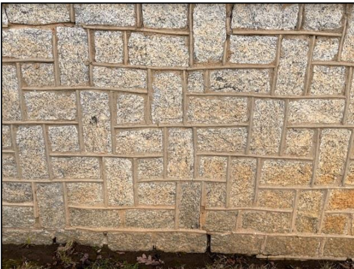
143. Typical minor cracks
