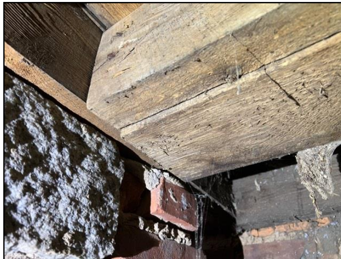
172. Poor end bearing, joist hanger connections
