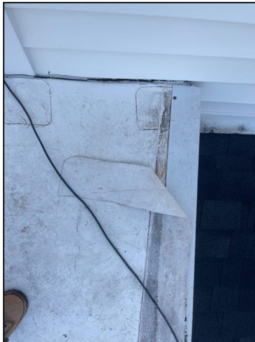
3. Openings at seams or flashings
