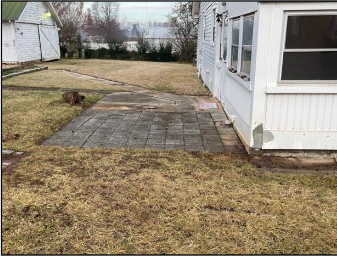
76. Improper slope or drainage
