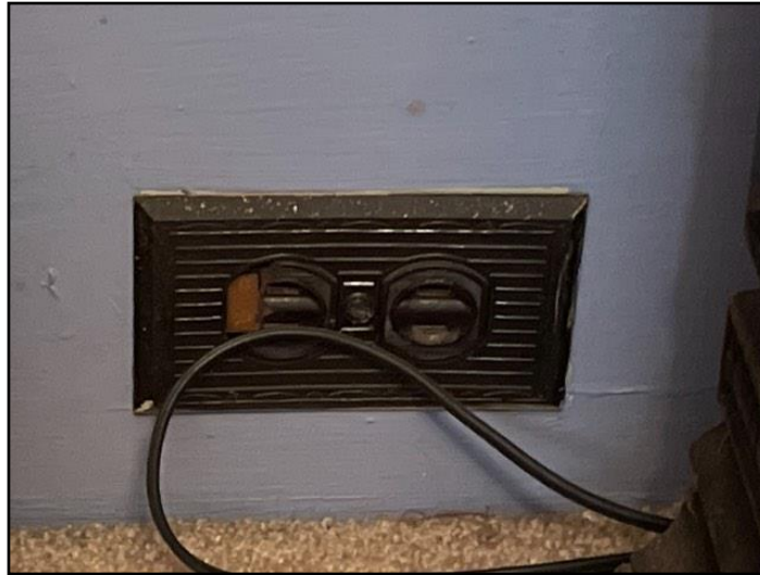
216. Damaged Outlet
