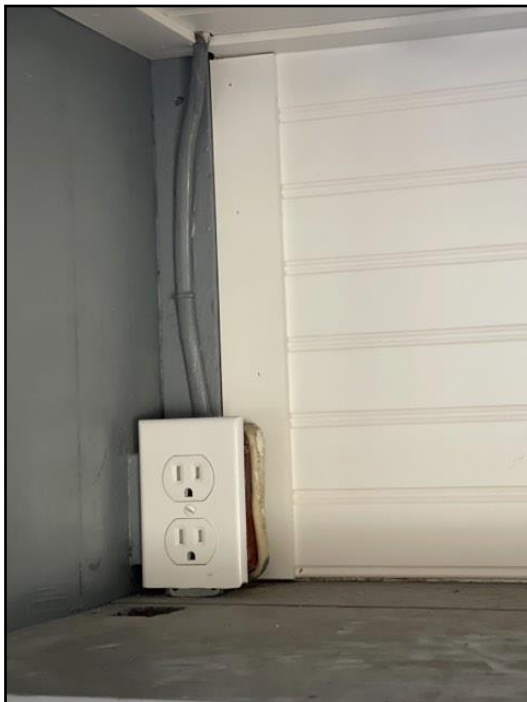
212. Exposed Electrical Wiring
