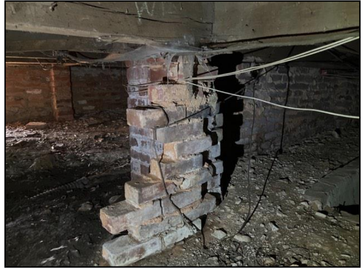
142. Poorly secured footing
