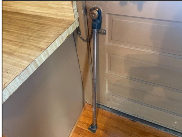
269. Lock not effective on exterior door
