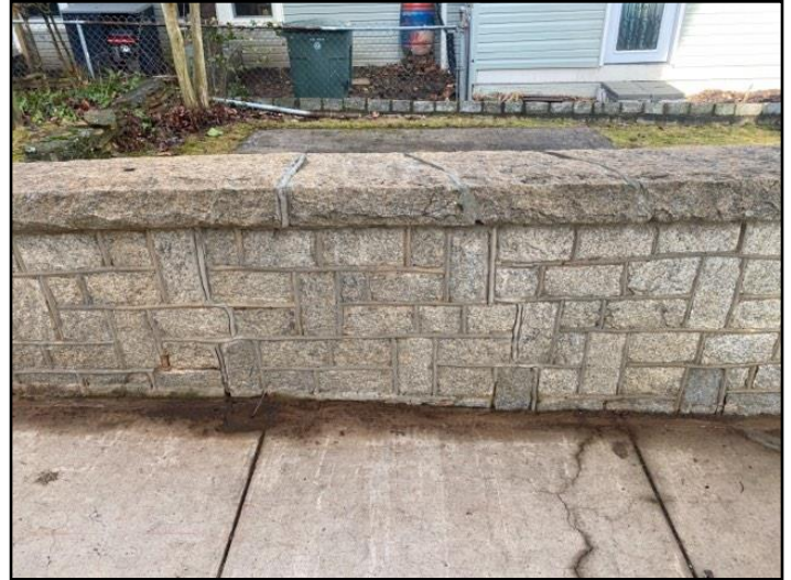
130. Patched Cracks
