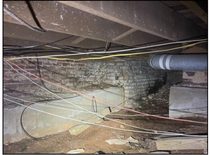
277. Efflorescence
