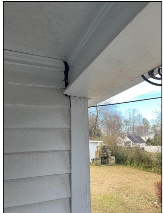
151. Movement caused by foundation movement
