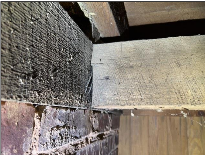
161. Poor bearing, crushed or loose shims
