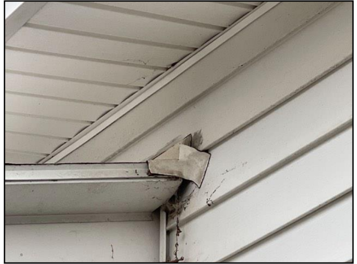
2. Openings at seams or flashings
