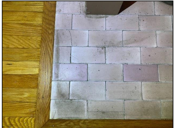
235. Gaps or cracks
