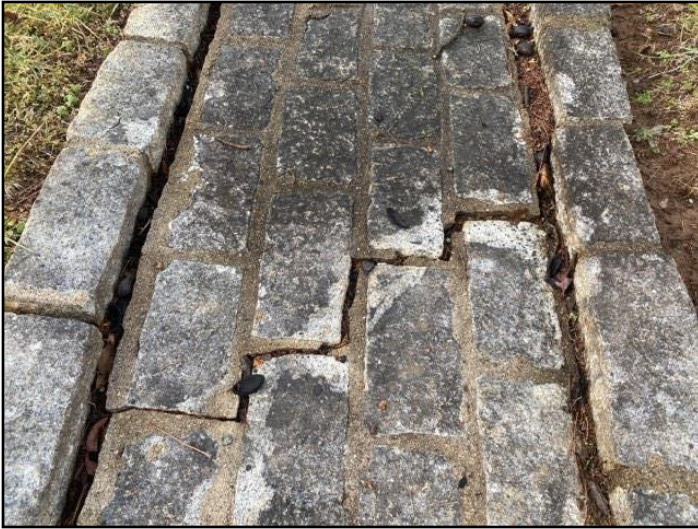
87. Cracked or damaged surfaces
