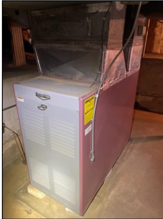
218. Oil Furnace (Basement)
