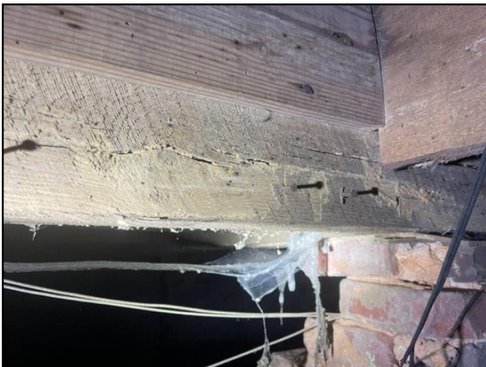
157. Evidence of wood destroying insects.
