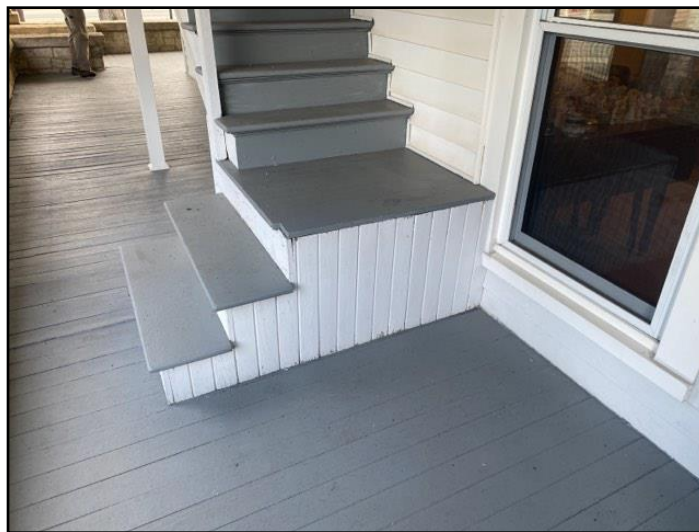
70. Missing Hand and Guardrail
