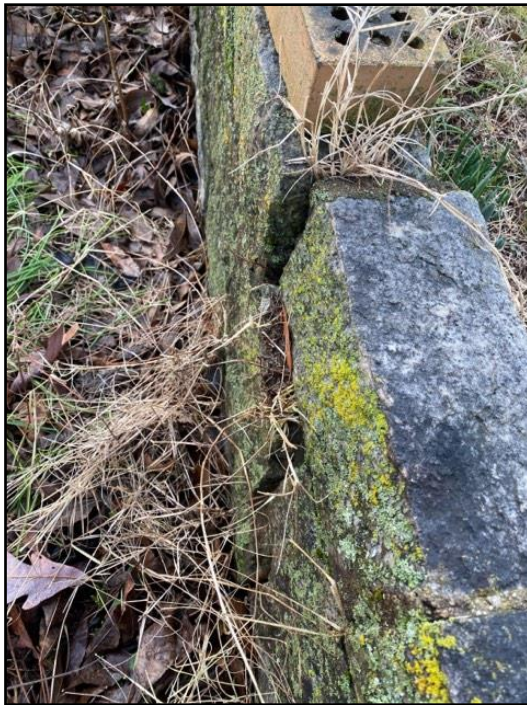
115. Settling or shifting
