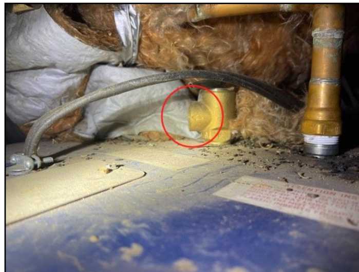
246. Discharge tube missing
