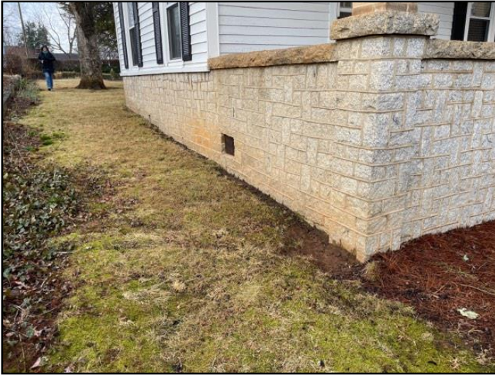
80. Improper slope or drainage
