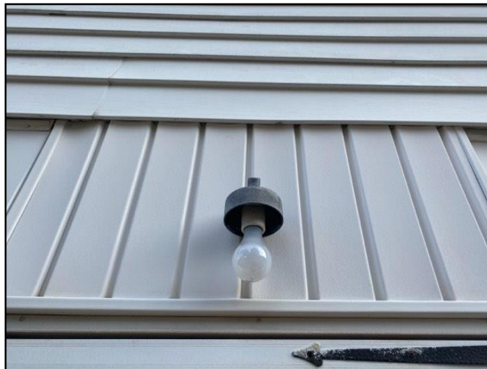
217. Light fixture globe is missing.
