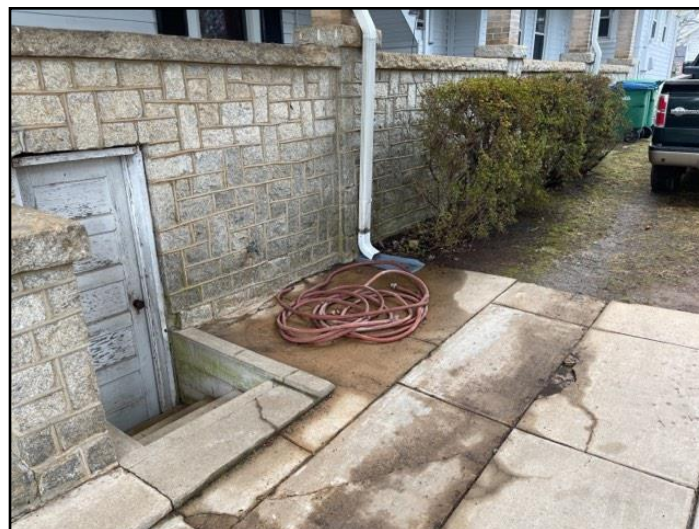
82. Improper slope or drainage
