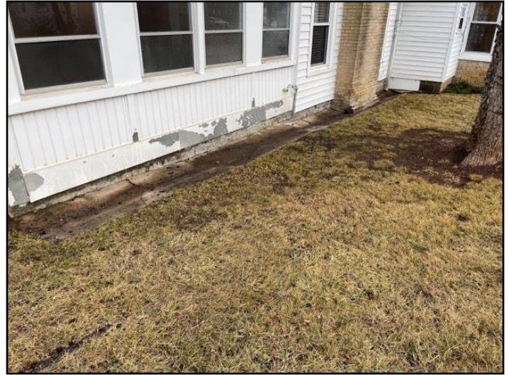
77. Improper slope or drainage
