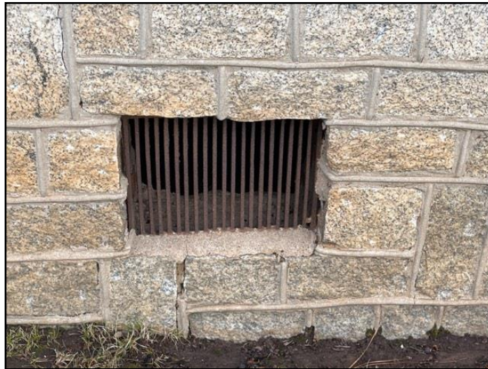
236. Damaged foundation vent screens....
