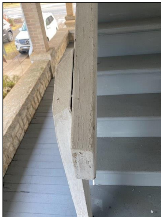
73. Handrail hard to hold.
