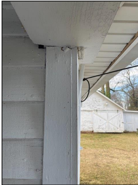
152. Movement caused by foundation movement
