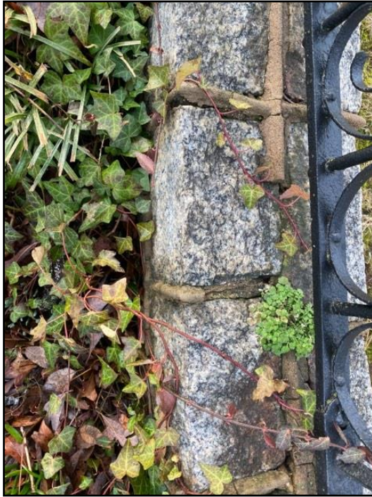
121. Mortar - deteriorated, missing
