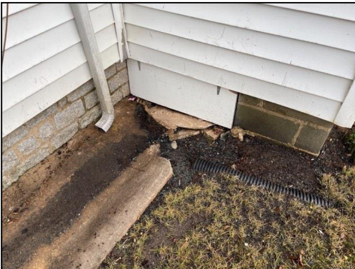
78. Improper slope or drainage
