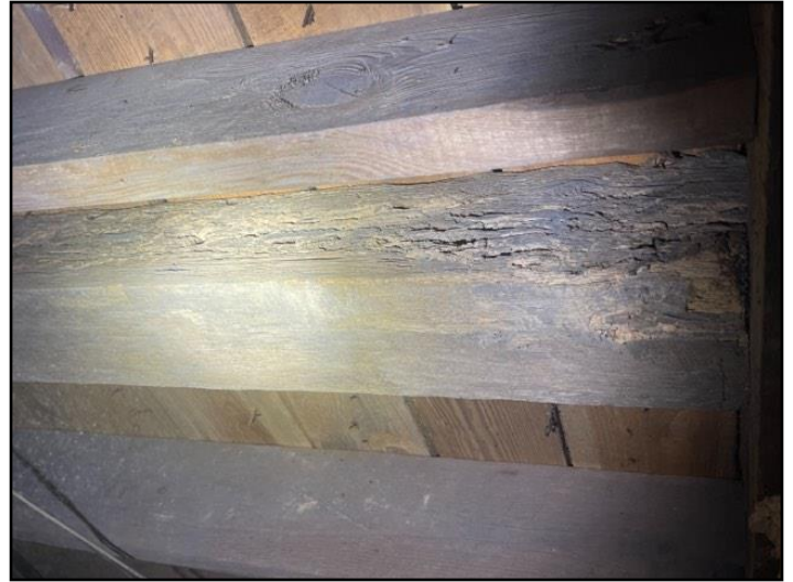
160. Evidence of wood destroying insects.
