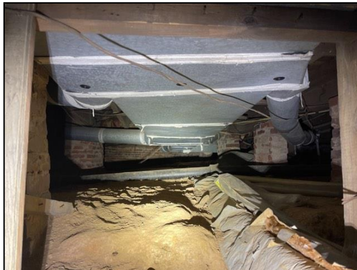
230. Exposed joint tape on the furnace...
