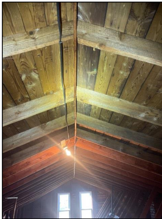
195. Undersized Ridge Beam - Properly sized ridg...
