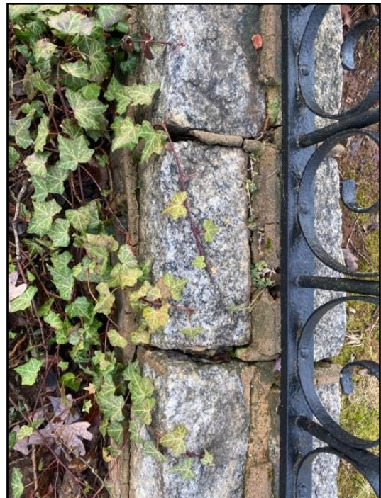
120. Mortar - deteriorated, missing
