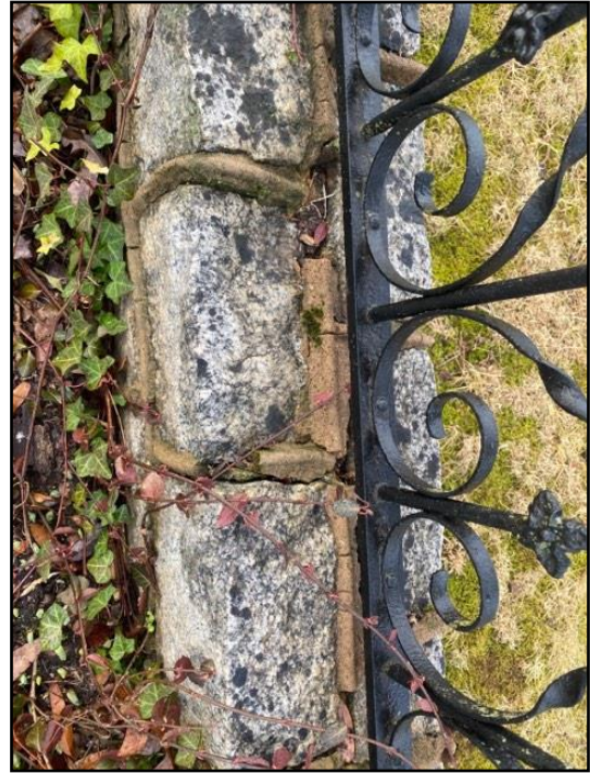
122. Mortar - deteriorated, missing
