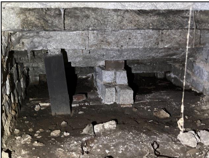
64. Inadequate support for stair - stair...
