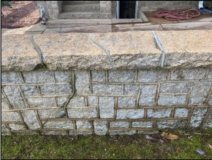
129. Patched Cracks
