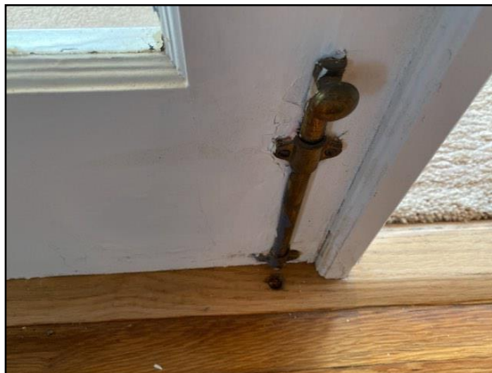
270. Does not latch properly
