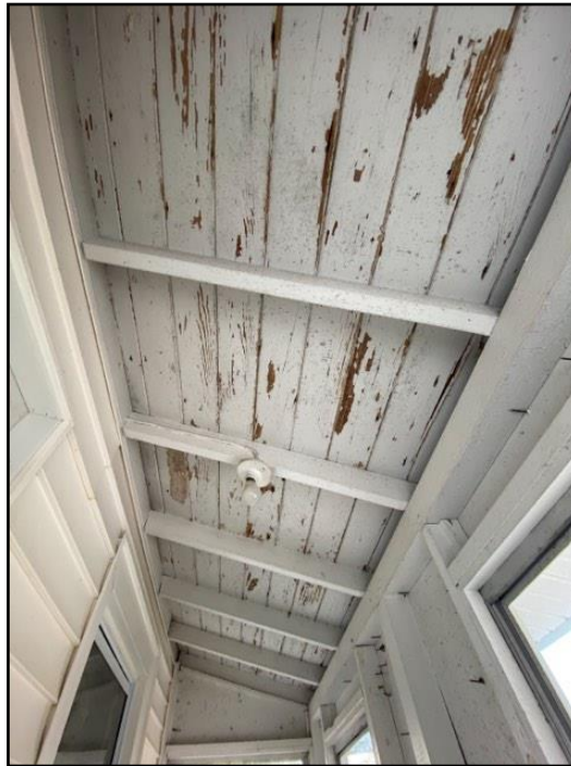
23. Paint - deteriorated / missing
