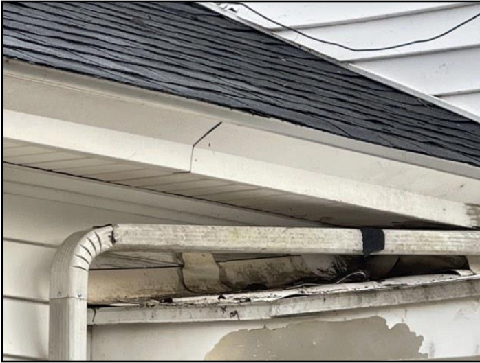
1. Openings at seams or flashings
