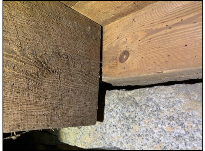
171. Poor end bearing, joist hanger connections
