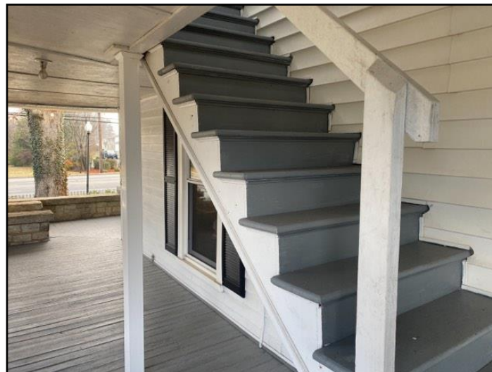
72. Spindles (balusters) missing
