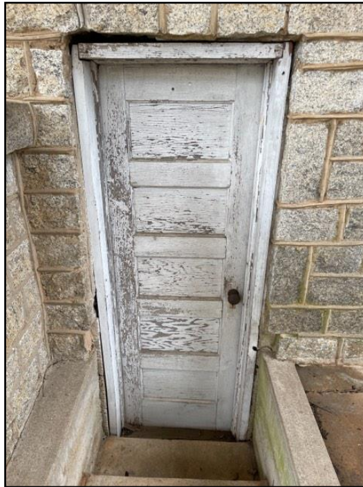
264. Weatherstripping missing or ineffective
