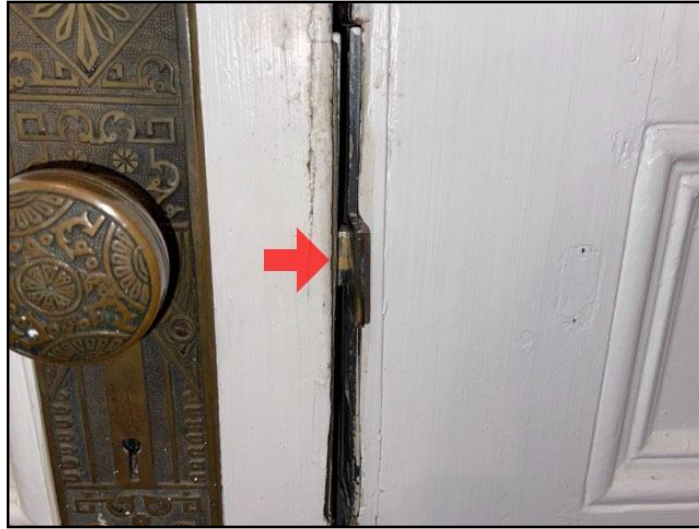
265. Over wide jamb margin at door latch
