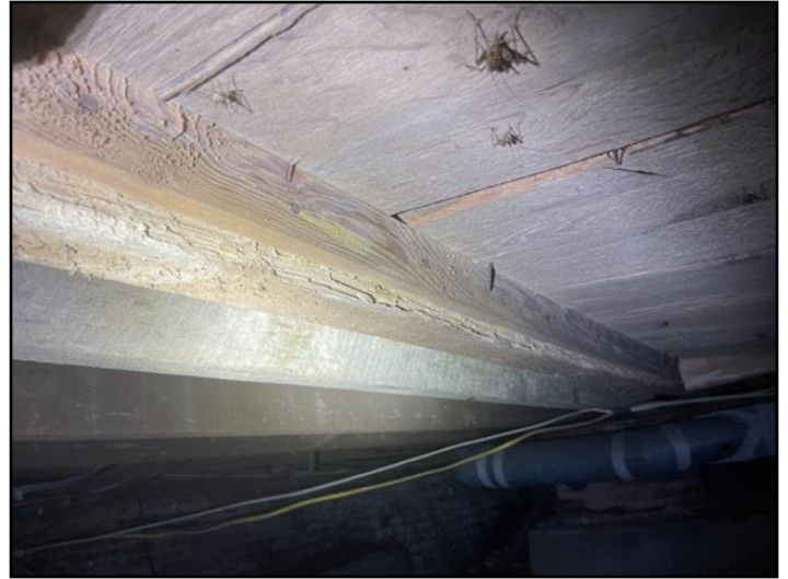
156. Evidence of wood destroying insects.
