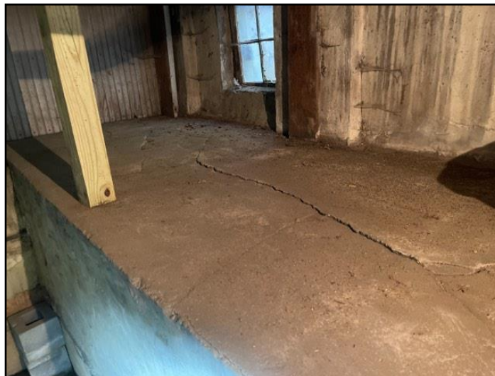
147. Typical minor cracks
