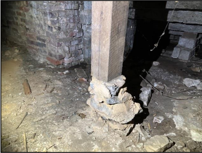
141. Poorly secured footing
