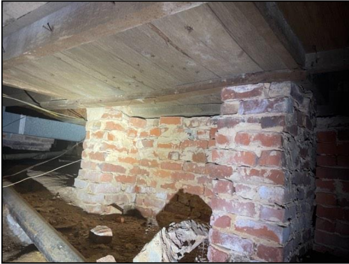
170. Poor end bearing, joist hanger connections
