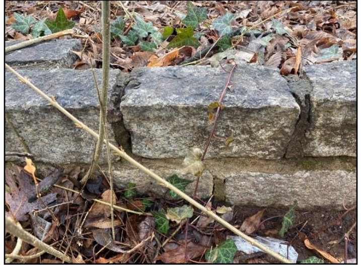
118. Mortar - deteriorated, missing
