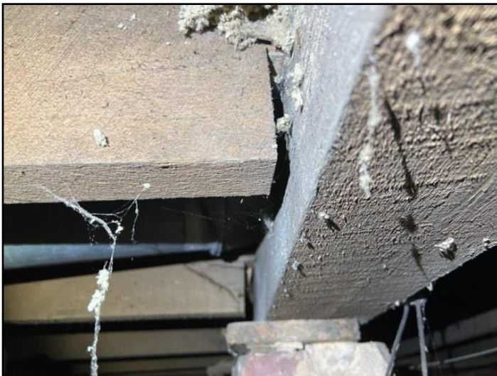
168. Poor end bearing, joist hanger connections
