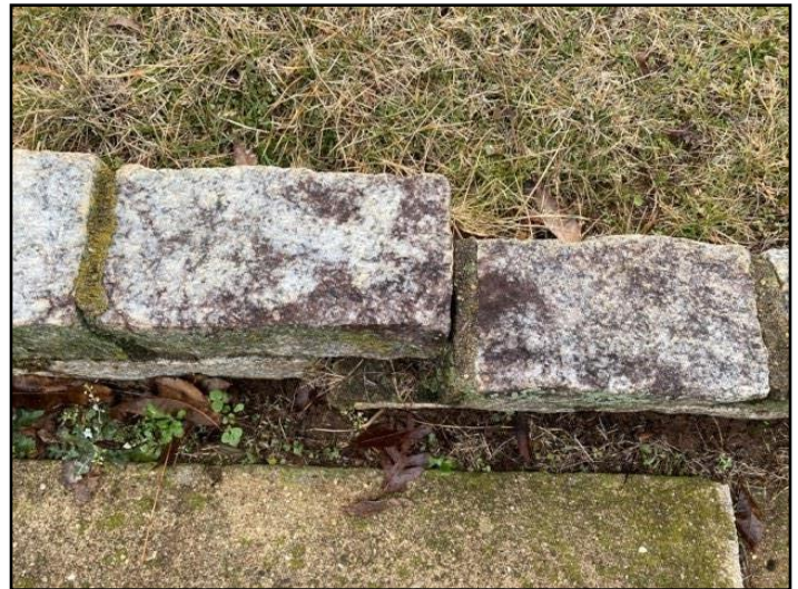
116. Settling or shifting
