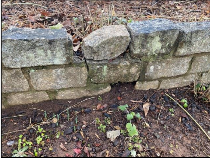
117. Mortar - deteriorated, missing
