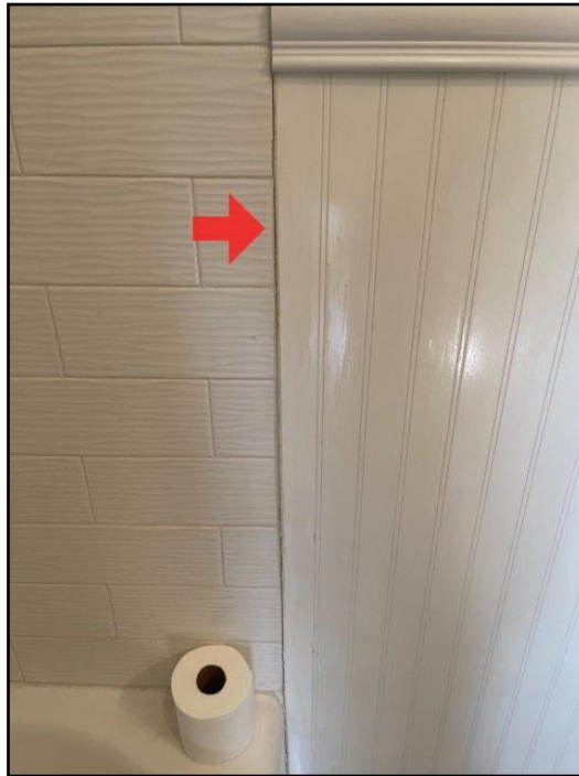
252. Caulking loose, missing or deteriorated
