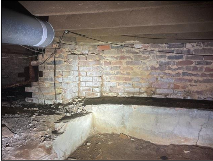
276. Efflorescence
