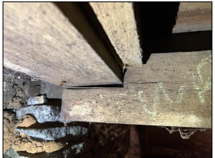
162. Poor bearing, crushed or loose shims
