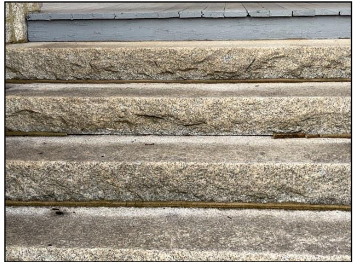
63. Missing or deteriorated mortar should be...
