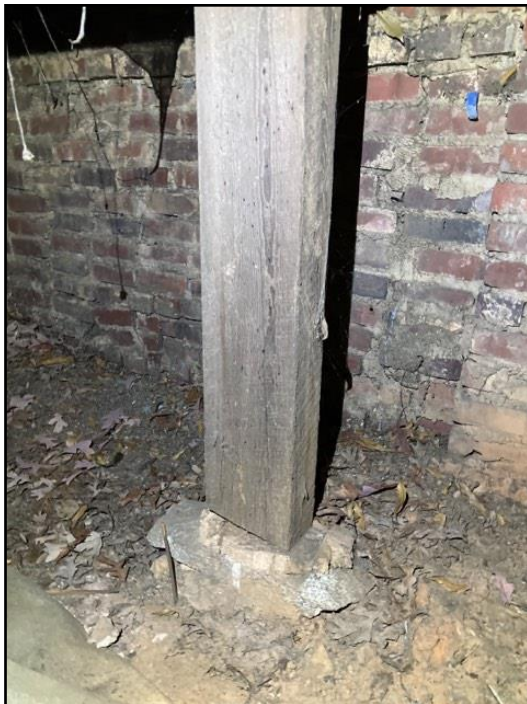
139. Poorly secured footing
