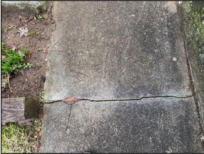
83. Cracked or damaged surfaces
