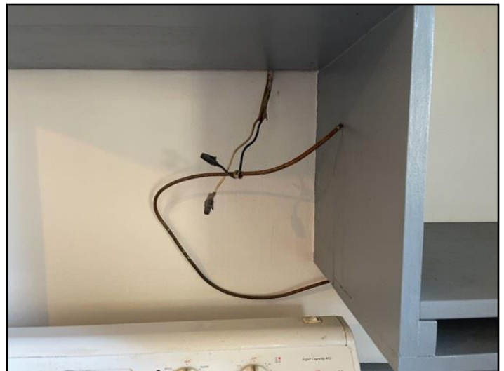
213. Exposed Electrical Wiring
