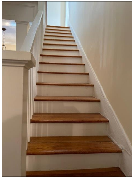
273. Missing Handrail
