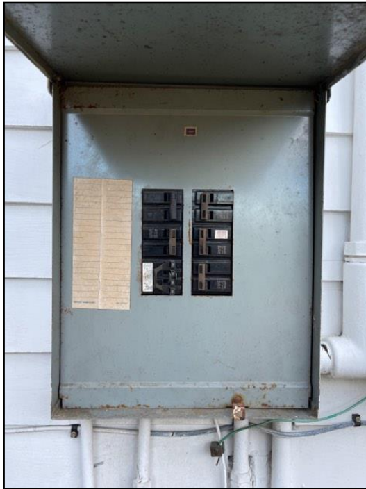
200. Main Electrical Distribution Panel
