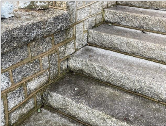
62. Missing or deteriorated mortar should be...
